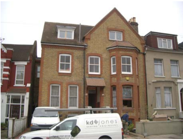
COMPLETED PROJECT VANT ROAD, WANDSWORTH
